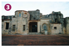
3 Iglesia de las Mercedes. Constructed between 1549 and 1555, the church was dedicated to the Lady of Mercedes.
