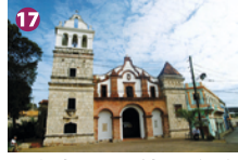
17 Iglesia de Santa Bárbara. Though date of construction is unknown, estimates point to the late 16th century. It was rebuilt after an earthquake in 1751.
